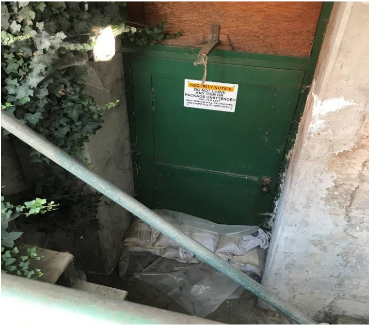
Figure 2-5 Basement Sandbags to Prevent Water Intrusion from Flooding – 75 Court Street
