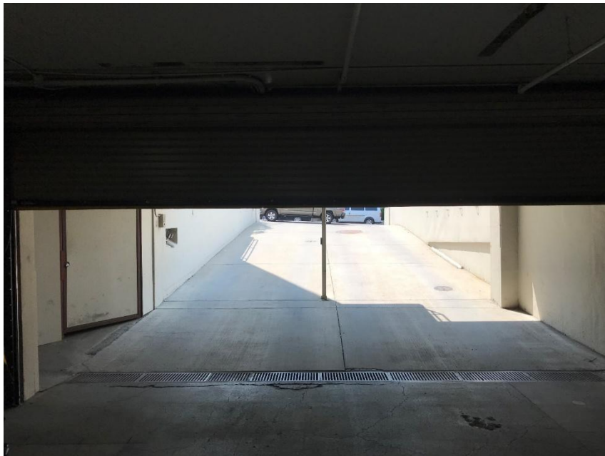
Photo of Entry Point into Basement Secure Garage – 75 Court Street
